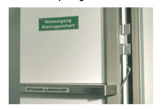
By using the integrated key switch, an authorised person may deactivate the e-Bar® in order to pass the emergency exit for a longer period of time. This status is communicated by a pulsating green display
