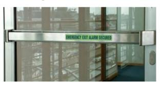
The emergency exit is in an alarm secured mode, which is indicated by a permanent green illumination when wired.
